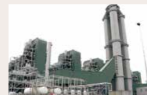
Kansai Electric Power Co., Inc.'s Himeji No. 2 Power Station (Construction - maintenance)
