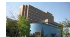
Techno Center (Sanda City, Hyogo Prefecture)
