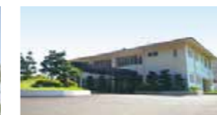
Nuclear Technology Training Center (Takahama Town, Fukui Prefecture)
