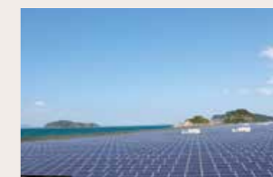
Arida Solar Power Station, Wakayama Prefecture (New construction work)
