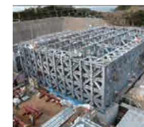
Tornado protection installation for seawater pump
