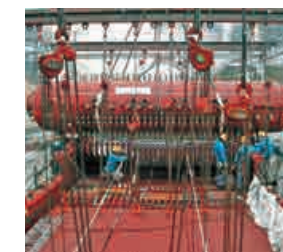
Steam drum installation, Tanigawa Mill, Hyogo Pulp independent power generation system
