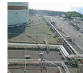
Temporary pipeline for tank cleaning
