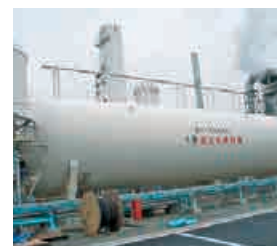
Liquid hydrogen tank and auxiliaries installation, Hydro Edge
