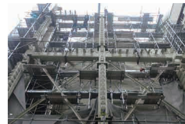
Tornado protection installation for condensate tank
