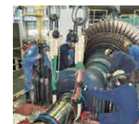
Turbine maintenance and overhaul, Himeji No. 2 Power Station, KEPCO
