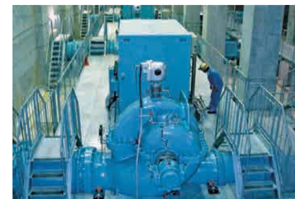
Water treatment pump installation
