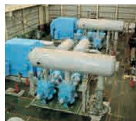
Boil-off Gas (BOG) compressor installation, Sakai LNG
