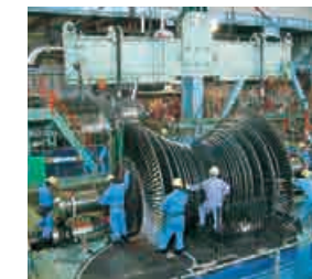
Steam turbine disassembly, Mihama Power Station, KEPCO
