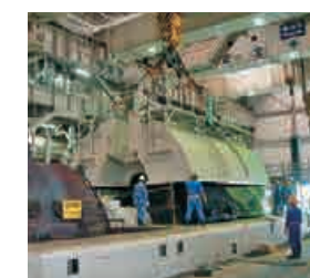
Turbine maintenance and overhaul, Nanko Power Station, KEPCO
