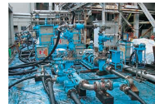
Temporary pipeline for boiler cleaning
