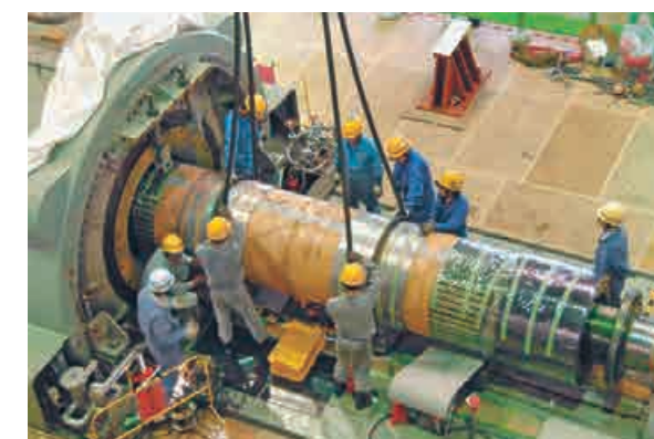
Electrics and generator rotor pull-out maintenance and overhaul, Aioi Power Station, KEPCO
